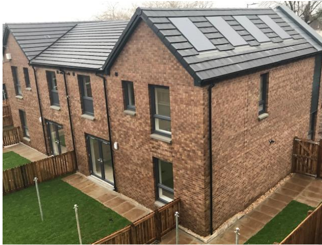
Sanctuary's Dubbs Road development, Port Glasgow
