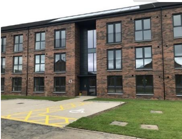
River Clyde Homes' St Stephens development, Port Glasgow
